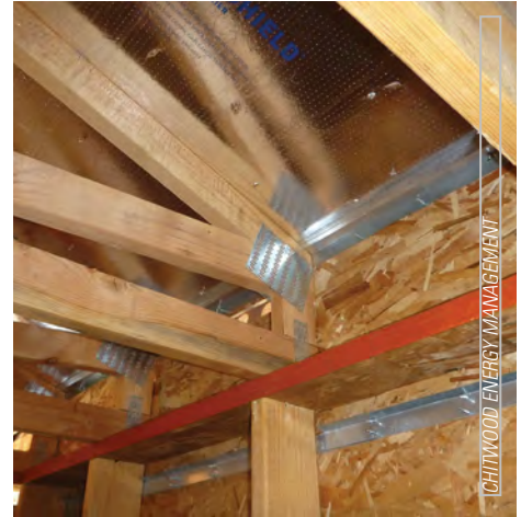
Raised Heel Truss detail, Habitat for Humanity, Dream Creek Subdivision, Stockton, CA. Designed by George H. Koertzen, Habitat for Humanity San Joaquin County, CA
